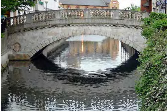
Bridge - Moulsham, Chelmsford, Essex
